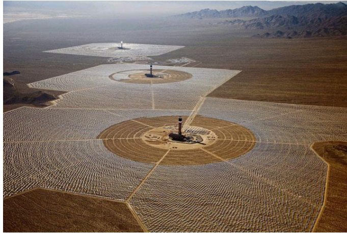
Ivanpah Solar Thermal Plant (3 units) 400 MWe total ( 25% Capacity Factor ) 37.5 m 2 /kWe
