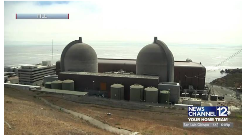
Diablo Canyon Nuclear Power Plants (2 units) 2256 MWe total ( 90% Capacity Factor ) 1.3 m 2 /kWe
