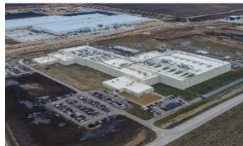
existing factories and chemical plants
